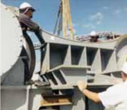
the driven rollers and the kiln tyre. The supporting rollers therefore have to compensate for the negative results of a thermally distorted kiln shell or foundation settlement without affecting the stability of the kiln support system.
